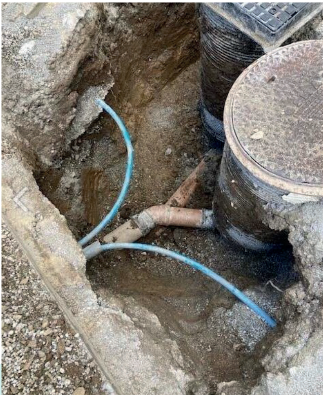
Left Illegal connection at manhole chamber (surface water MH has the circular cover)
